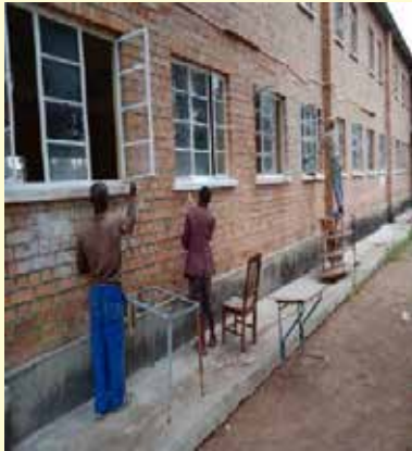
The refurbished windows have been sealed and now have locks, offering greater comfort and safety.
