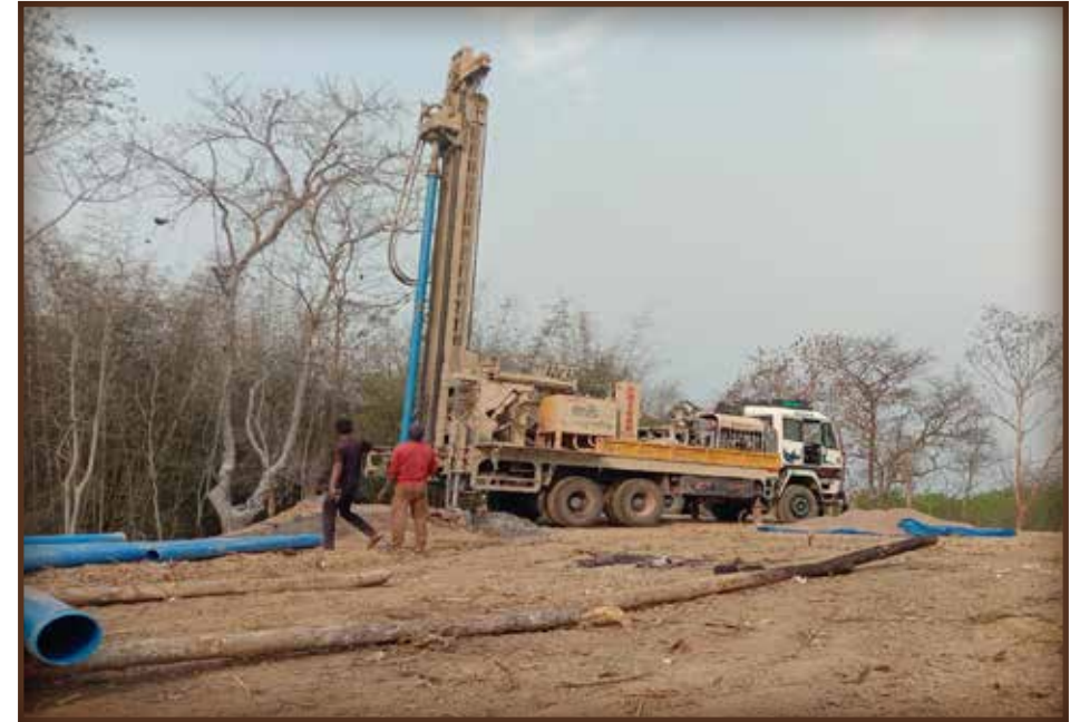
Foundations of Friary commence : Borewell Digging.
