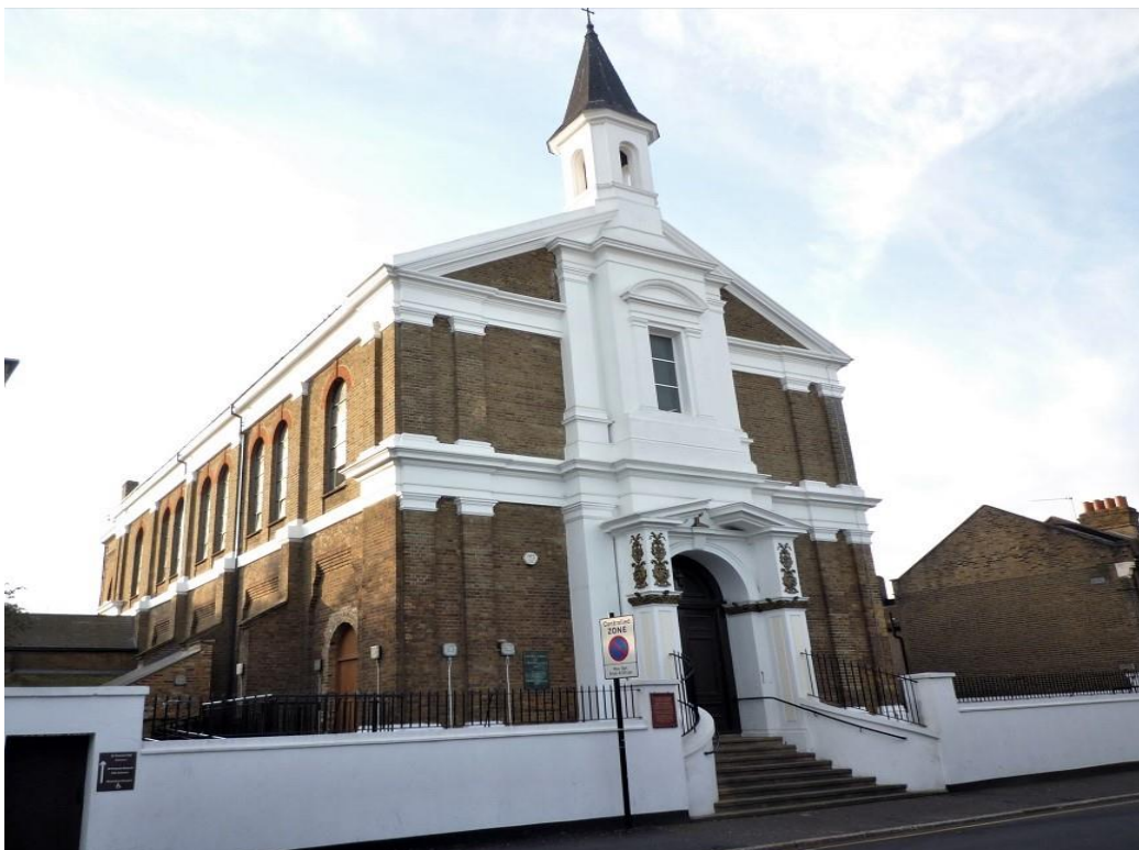
Figure 4 Church of St Francis of Assisi, Stratford
